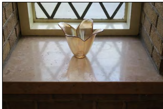
101 Kalkstenen vensterbank in centrale hal.
