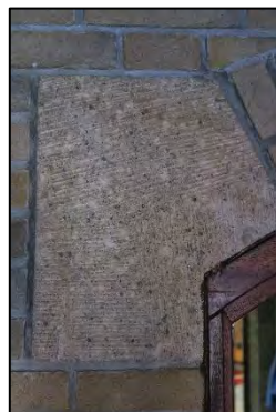
104 Gefrijnde stenen detaillering.
